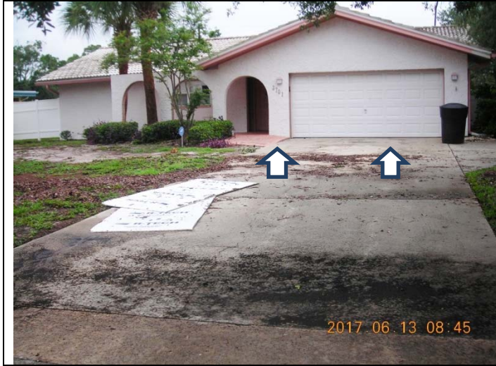
Flood Water Lines at 42 nd Ave./37 th St. S
