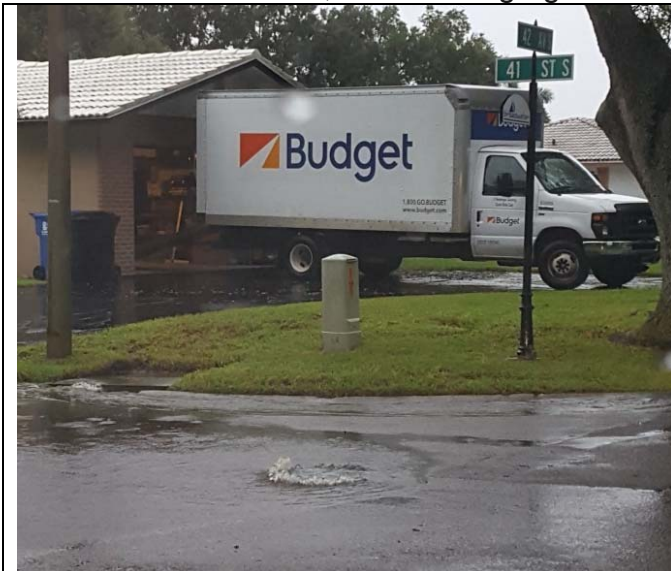
Overflowing Sanitary Sewer at 42 nd Ave./ 41 st St. S
