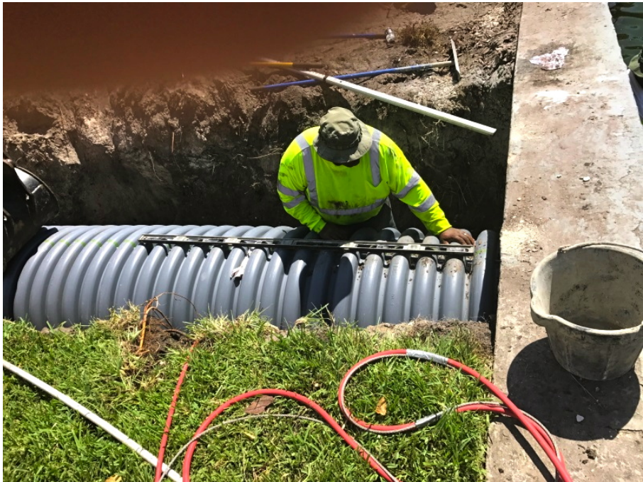
Connecting 36" drain to seawall at 42 nd Ave. S/39th St. S (photo courtesy Gerry Moore)
