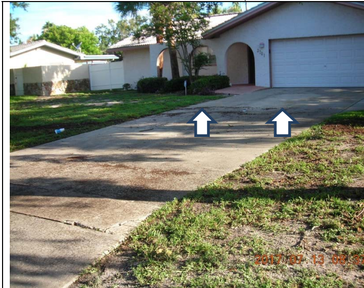
Flood Water Lines at 42 nd Ave./37 th St. S (same house 1 month later)
