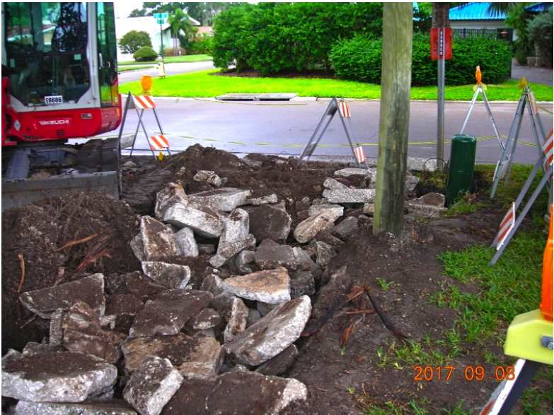
Interim connection to 42 nd Ave. S allowed functional draining of storm water during Hurricane Irma
