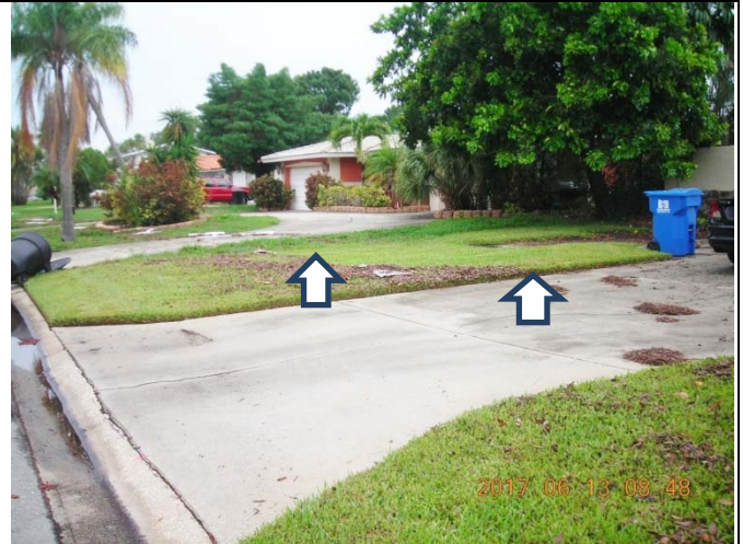
Flood Water Lines at Adjacent House on 42 nd Ave. S.
