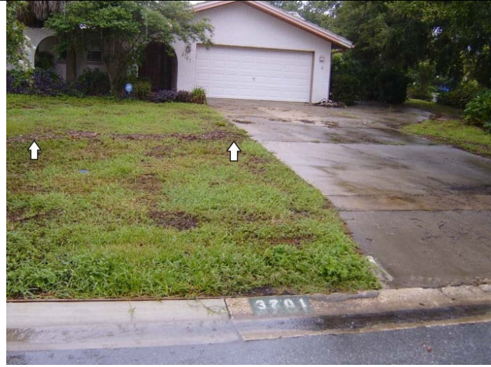
Subsequent Flood Water Lines at 3701 42nd Ave S
