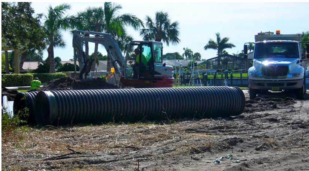
In-progress 42 nd Ave. S/41 st St. S drain
